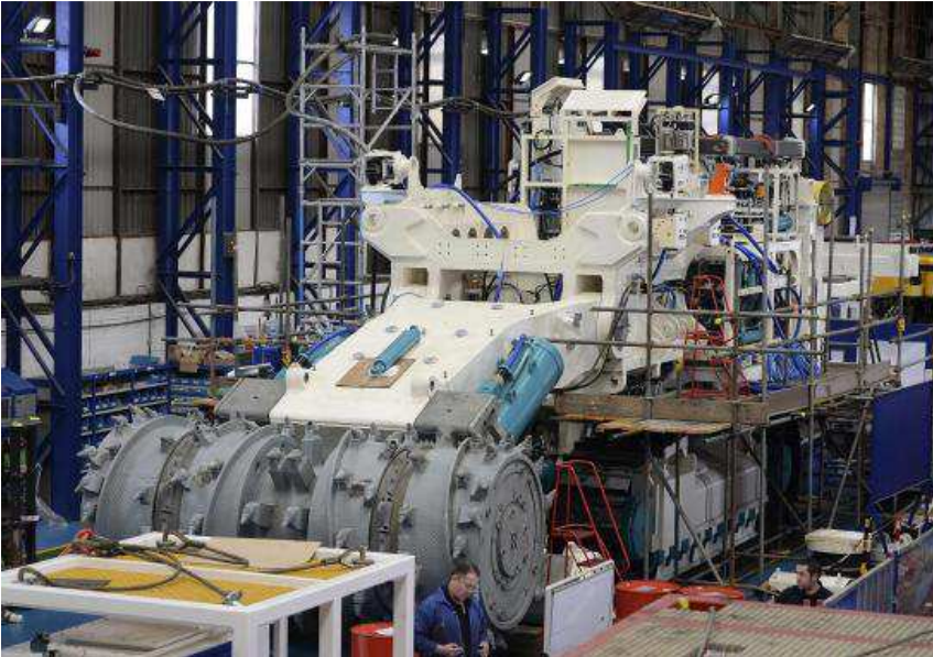
Employees of Soil Machine Dynamics (SMD) work on a subsea mining machine being built for Nautilus Minerals at Wallsend, northern England April 14, 2014. Credit: Reuters/Nigel Roddis
